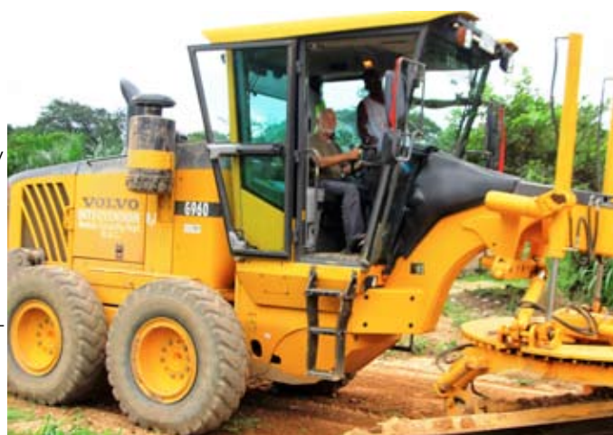
Road Improvement Project
