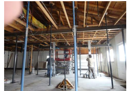
Repairing failed roof trusses in Bisbee
