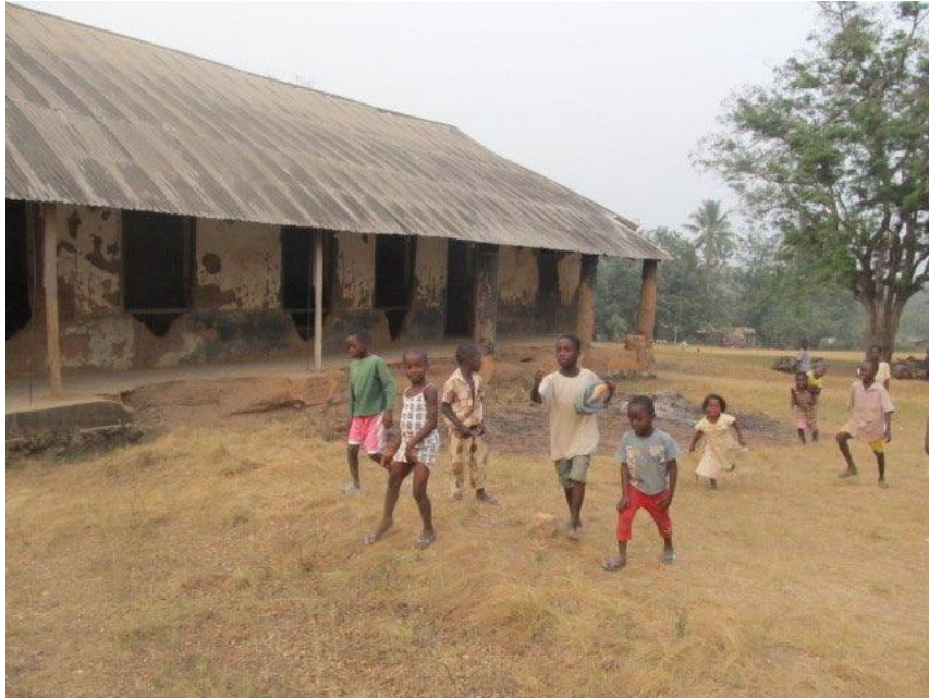
Bueman Community Multi-Purpose Learning Center Restoration Project
