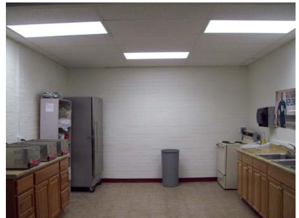
Manuel Bojorquez Learning Center Kitchen Remodel
