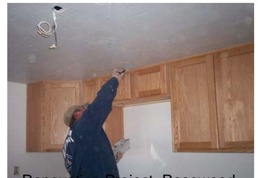
Renovation Project, Rosewood Group Home, Tucson
