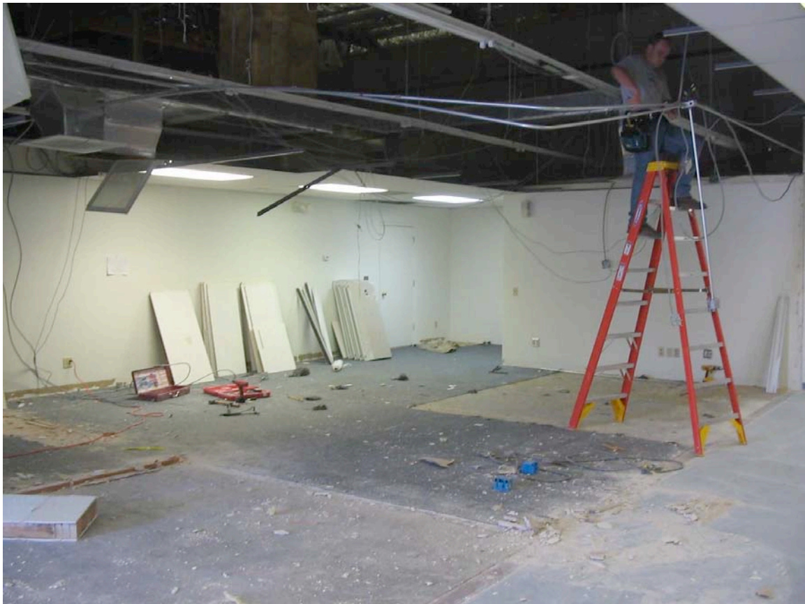
Cesar Chavez Hall of Fame During Construction
